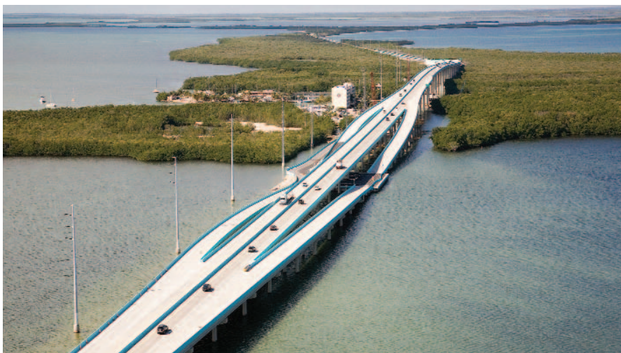
The Florida Dept. of Transportation will be making extensive use of design-build for its stimulus projects. (Photo courtesy Granite Construction Co.)
