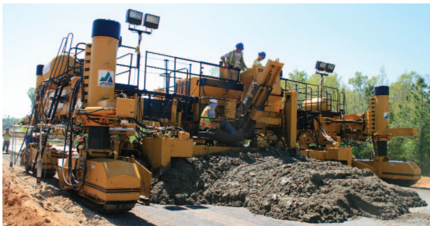
The $298 million in stimulus funds that will go to the Louisiana Dept. of Transportation and Development will create a statewide ripple effect. James Construction Group of Baton Rouge, La., paves two new lanes on US 167 in north Louisiana. (Photo by Sam Barnes)
